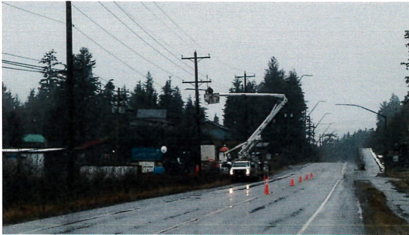
Three-phase service installation, North Tongass Hwy
