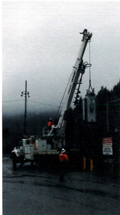
Installation of new pole & LED light over cross-walk at Valley Park school building on Schoenbar Road
